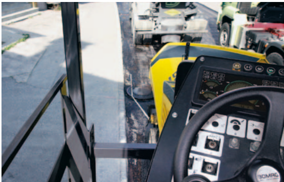
Unobstructed view onto the guide rod
