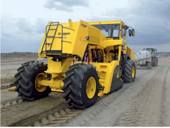
BOMAG MPH 600 on soil stabilisation ...
